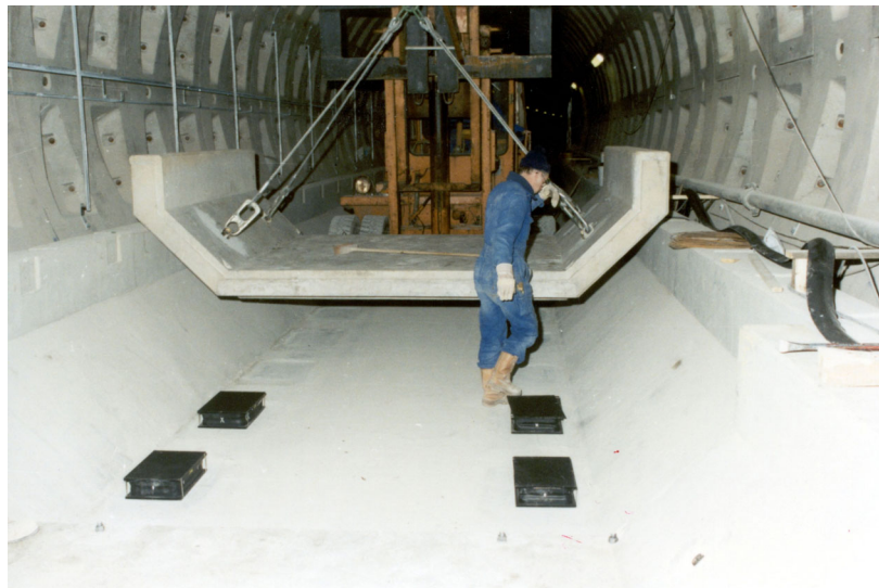
Figure 2.4: Installation of a floating-slab track in the form of precast reinforced concrete tray (courtesy of GERB, Germany [36]).
