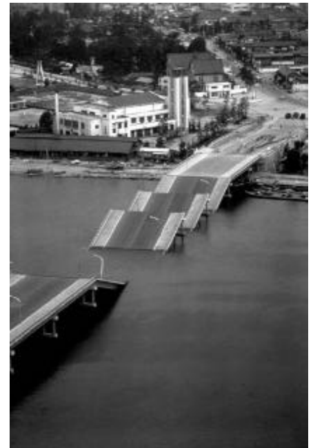
Figure 13 Collapse of the Showa bridge in the 1964 Niigata earthquake (after Hamada 1992).
