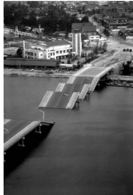
Figure 1. Collapse of the Showa bridge in the 1964 Niigata earthquake (after Hamada 1992).
